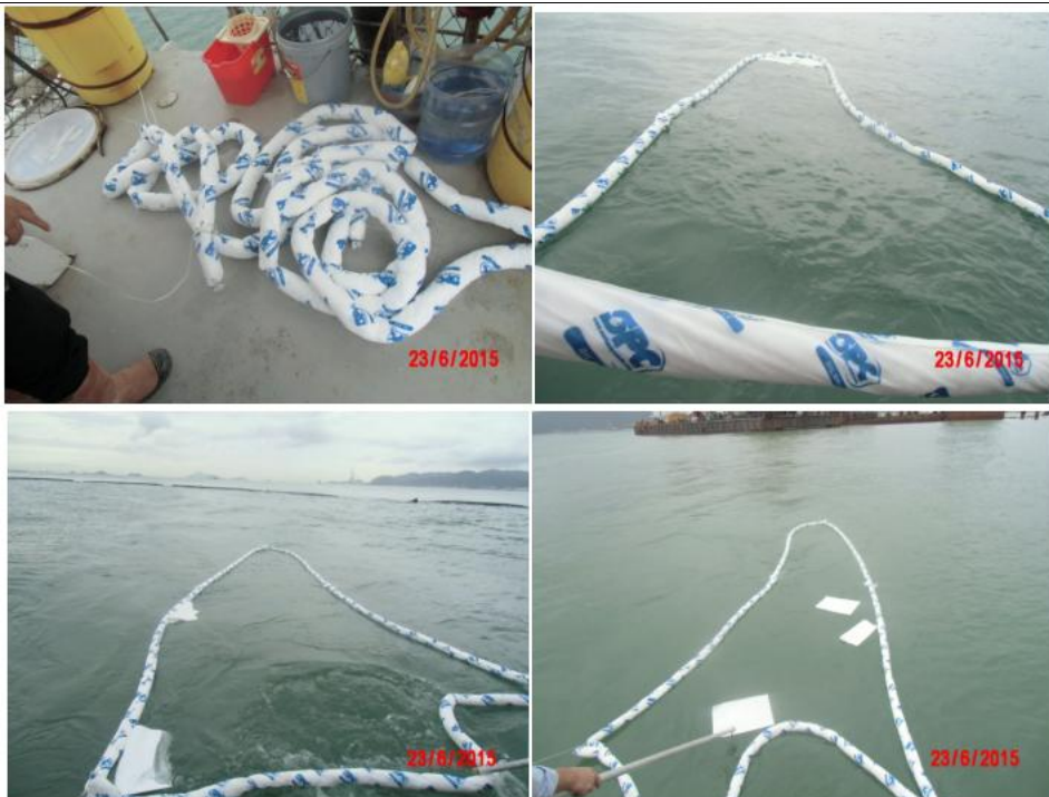
6.4.23 The used absorption booms were collected using disposal bags as part of the spill kits item. The used absorption booms were disposed of as chemical waste by the Contractor. (Also refer to photo record below)
