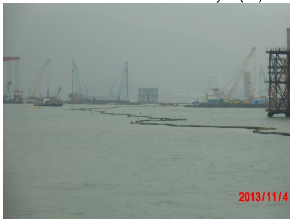
Photo record of site condition nearby IS(Mf)6
