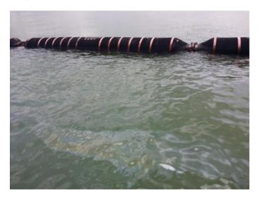
• The Contractor deployed absorption booms to remove the floating oil from water and the used absorption booms were collected using disposal bags as part of the spill kits item. The used absorption booms were disposed of as chemical waste by the Contractor. (Also refer to photo record below).
