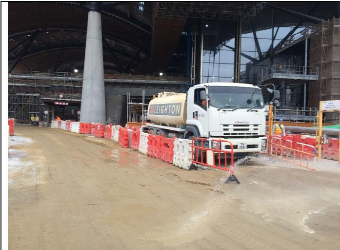
Water truck spray water on haul road (Point A)
