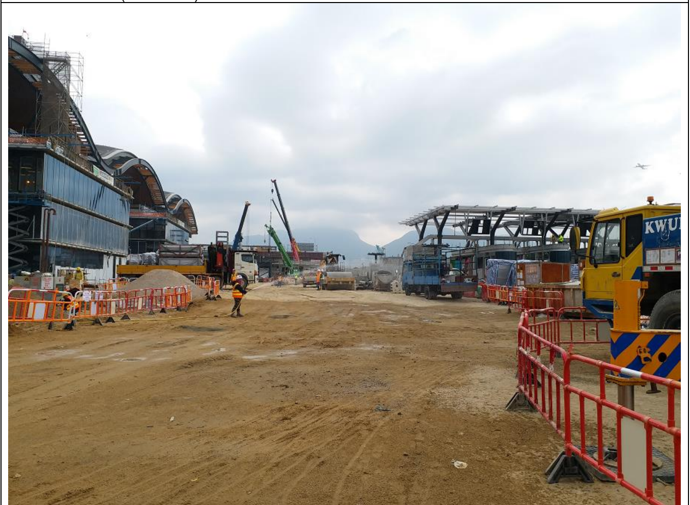
Water spray on haul road (Location 2)
