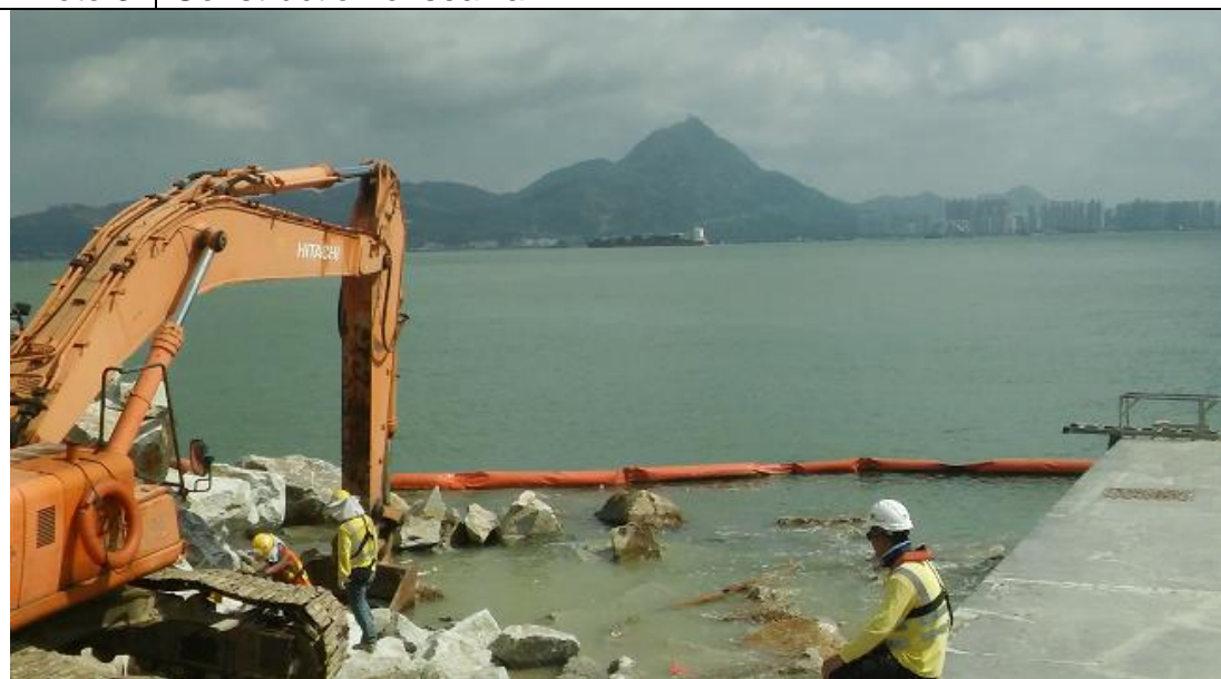
Photo 3 | Construction of seawall
