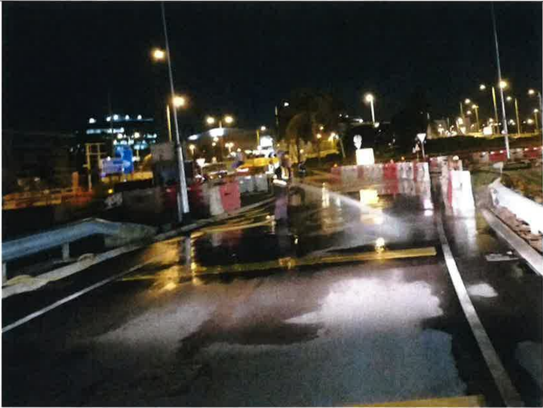
Photo 180312_001 – Photo taken on 12 March 2018 at the site exit
