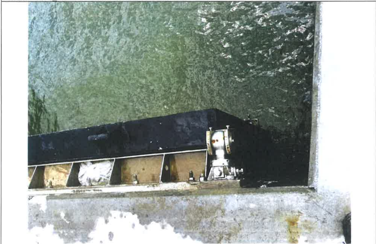
Photo 180627_002 -Box Culvert A on 27 June 2018
