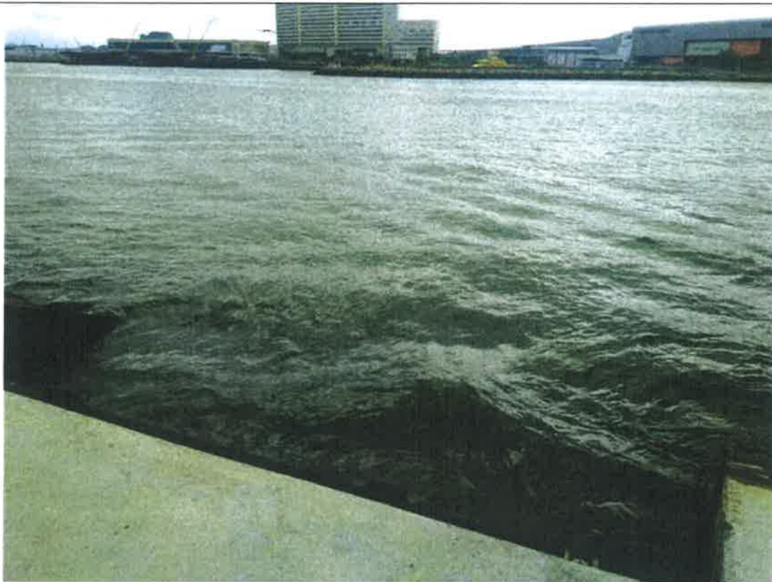
Photo 180625_001 –Box Culvert A on 25 June 2018
