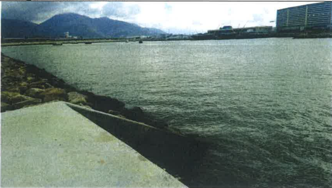
Photo 180625_002 –Box Culvert A on 25 June 2018
