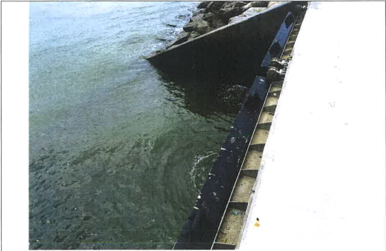
Photo 180627_001 -Box Culvert A on 27 June 2018
