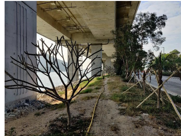
Description: General view of planted trees ( Plumeria rubra and Phoenix roebelenii )
