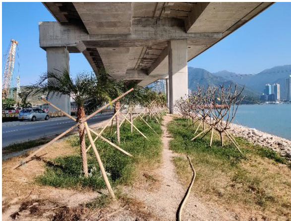
Description: General view of planted trees ( Plumeria rubra and Phoenix roebelenii )
