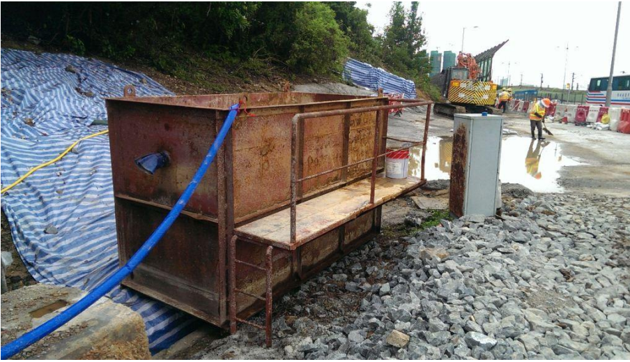
General mud and soil removal
