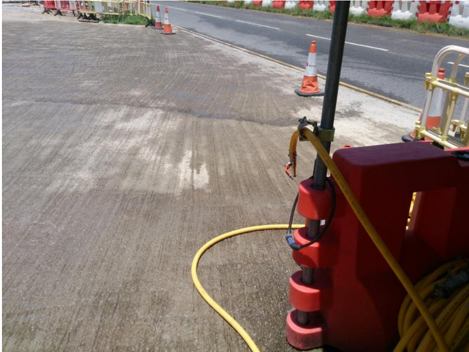
Wheel washing facility at Site Access 3B
