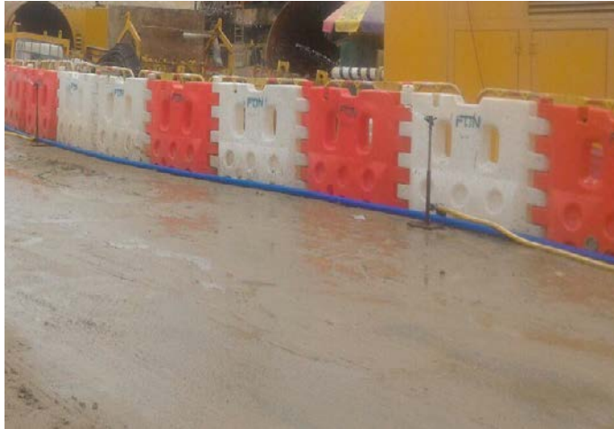
Photo 2 - Water sprinklers installed on the soil stockpile for dust suppression
