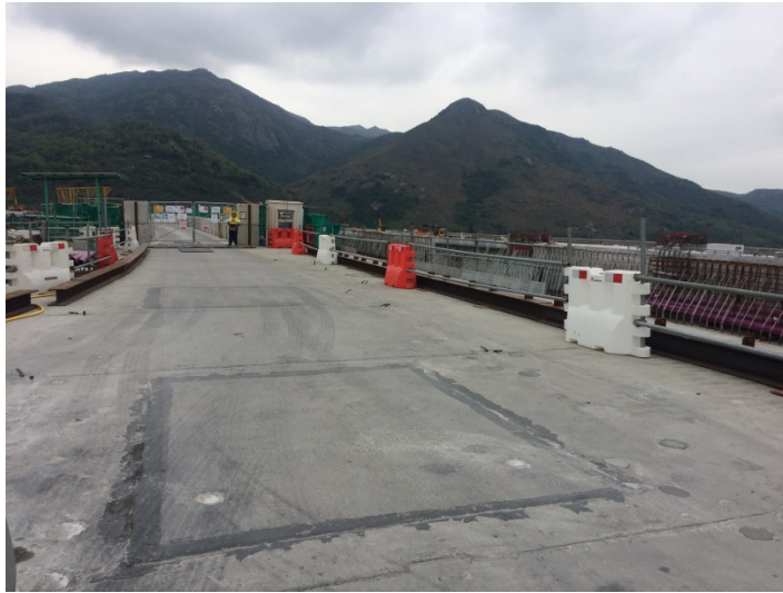
Photo 4 - High toe-board and erected guard-rails were installed between gaps
