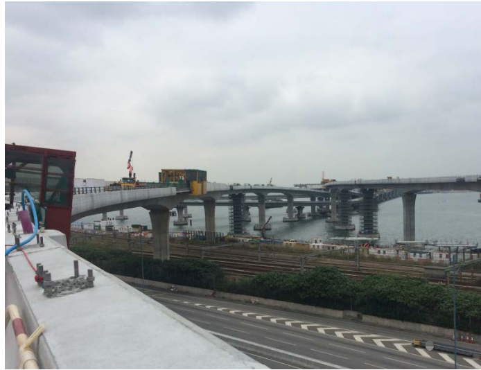
Photo 2 - Land portion of Viaduct B (near Tai Ho Wan)
