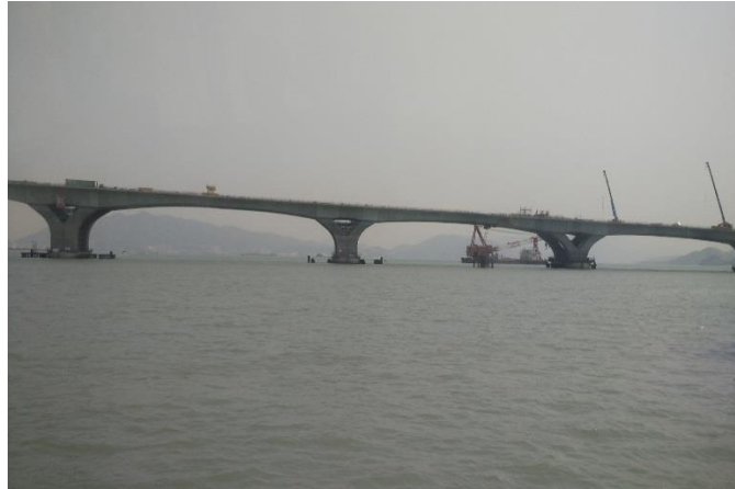
Photo 1 - Mid-Flood at IS8 on 23 March 2018
