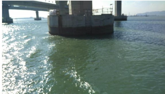
Photo 6 - Mid-Flood at SR4a on 8 August 2018
