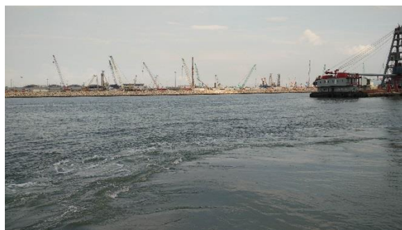
Photo 2 - Mid-Ebb at SR4a on 7 September 2018
