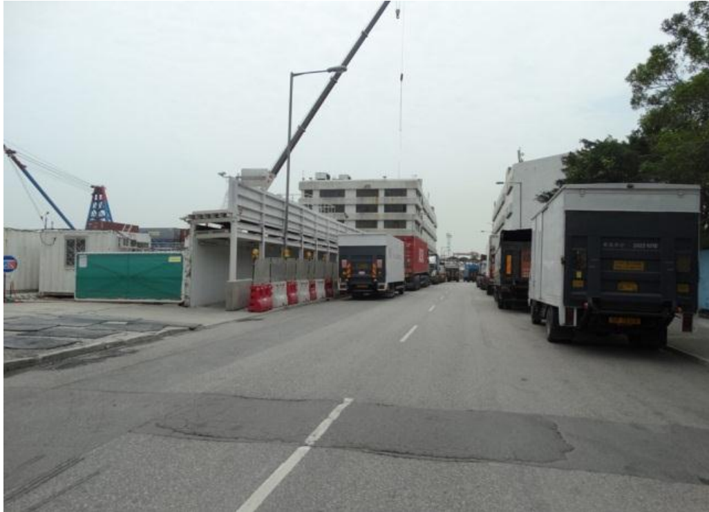
Site Entrance at Ho Yeung Street
