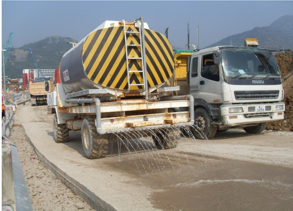
Water truck was observed in used during site investigation. (Reclamation Works Area)
