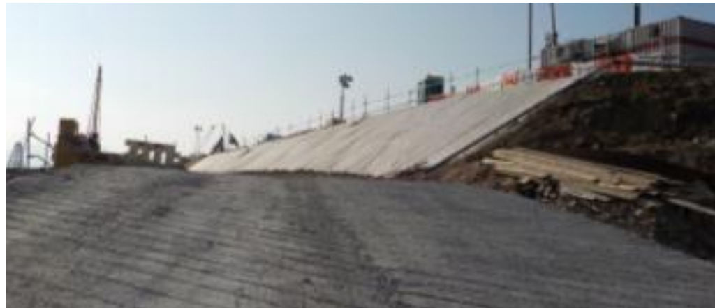
Hydroseeding and access roads paved as soon as practicable after works have been completed on soil exposed area. (Reclamation Works Area)
