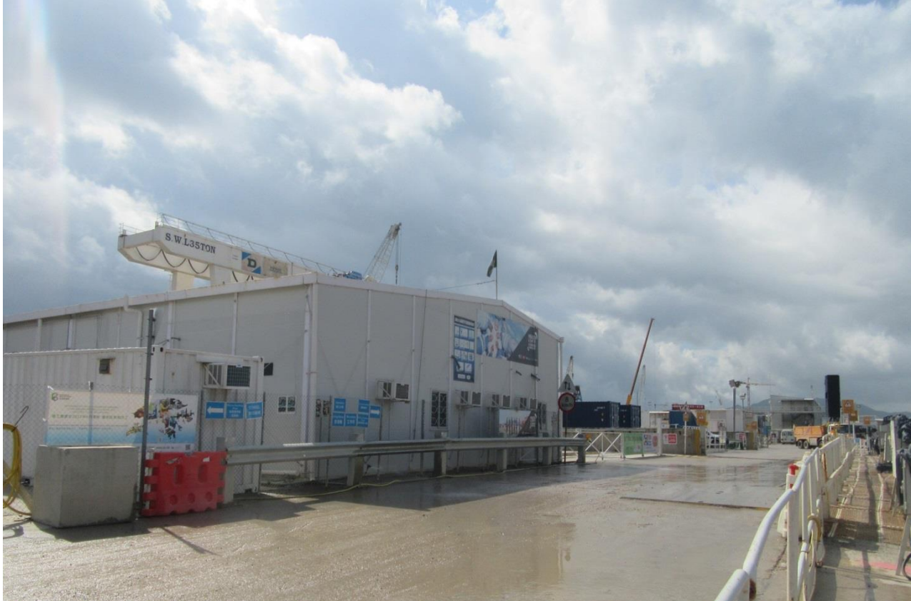
Water spraying was applied frequently during dry conditions.(Works Area Portion N-A)
