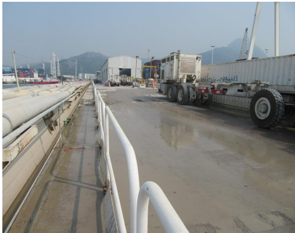
Sprinklers are installed for water spraying. (Works Area Portion N-C)
