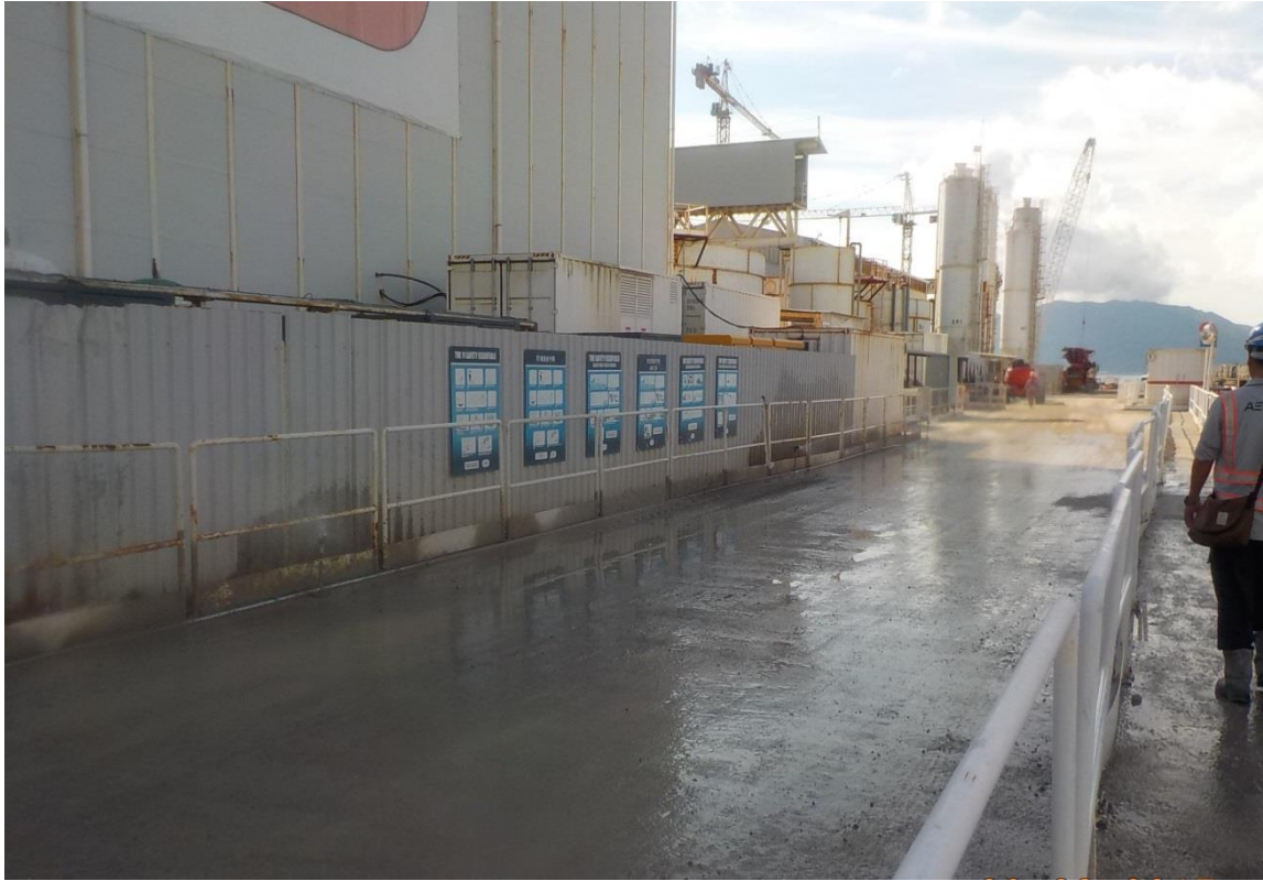
Water spraying was applied frequently during dry conditions.(Works Area Portion N-B)
