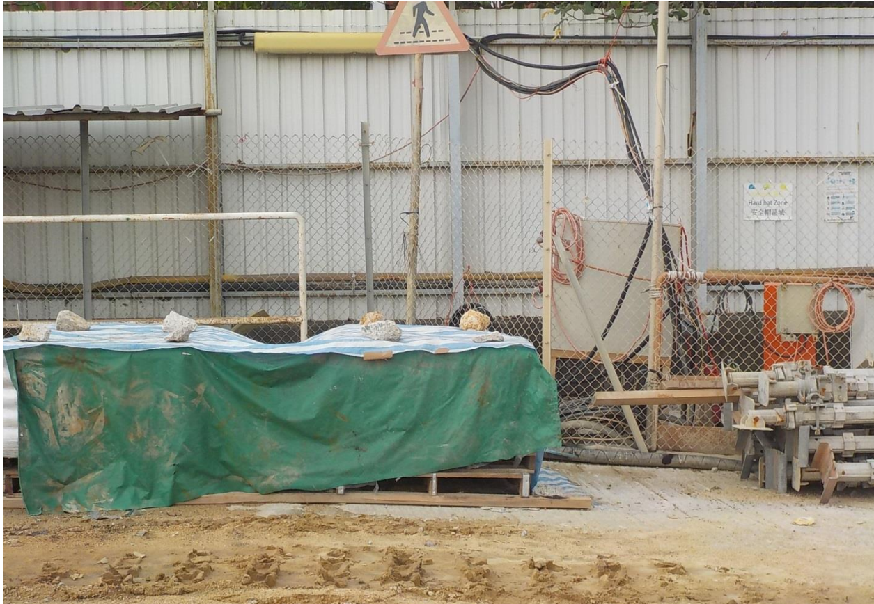
Cement bags are covered by tarpaulin sheets. (Works Area Portion N-A)
