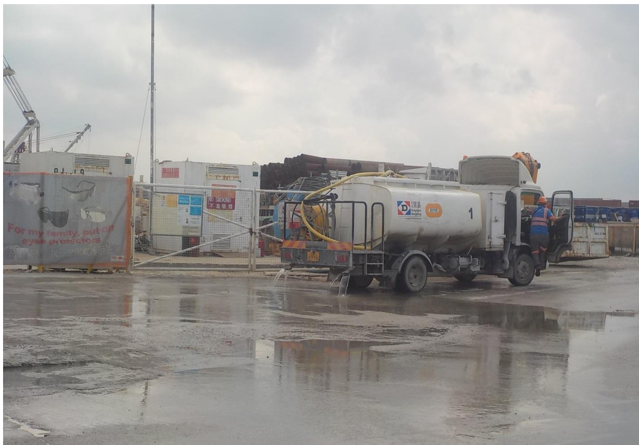
Use of water truck for water spraying. (Works Area Portion N-A)
