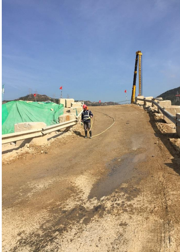
Water spraying was applied frequently on site. (Works Area Portion N-A)
