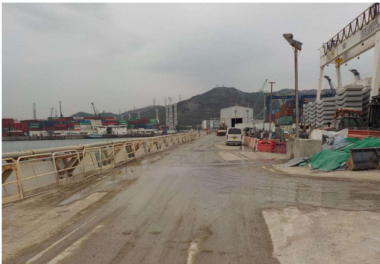
Water spraying was applied frequently on site. (Works Area Portion N-B)
