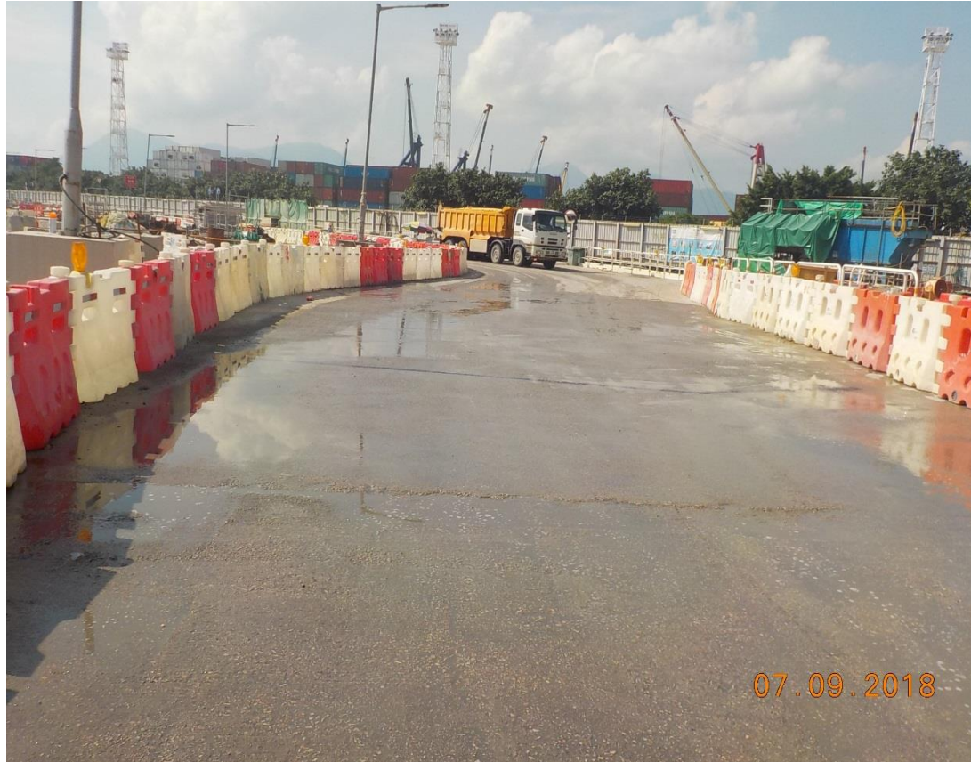
Water spraying was applied frequently on site. (Works Area Portion N-A)
