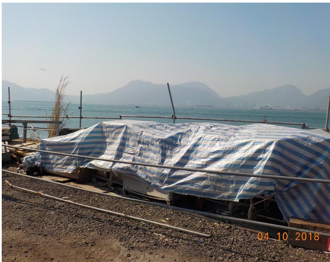
Dusty material was covered by tarpaulin sheet. (Works Area Portion N-C)
