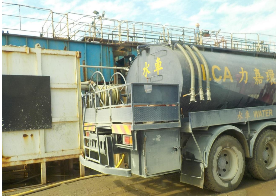
Water truck was used for dust control. (Works Area Portion N-C)
