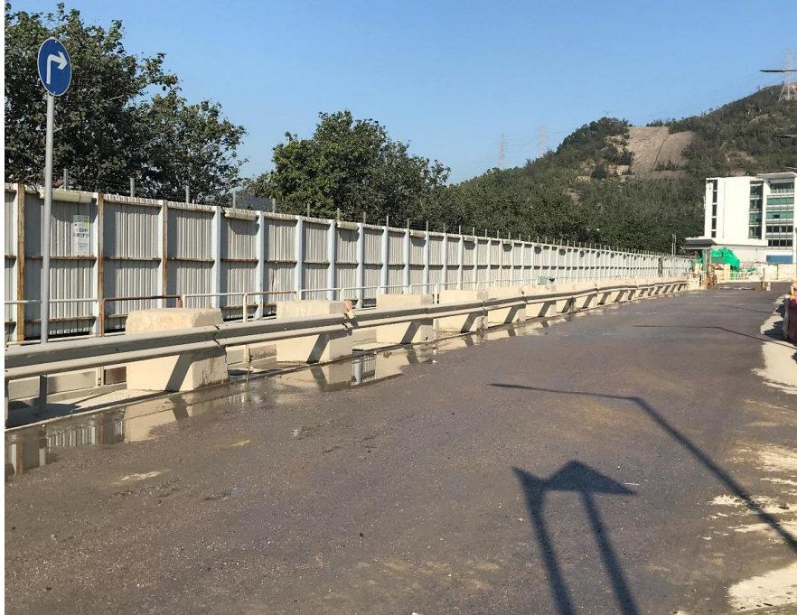
Water spraying was applied on the main haul road. (Works Area Portion N-A)
