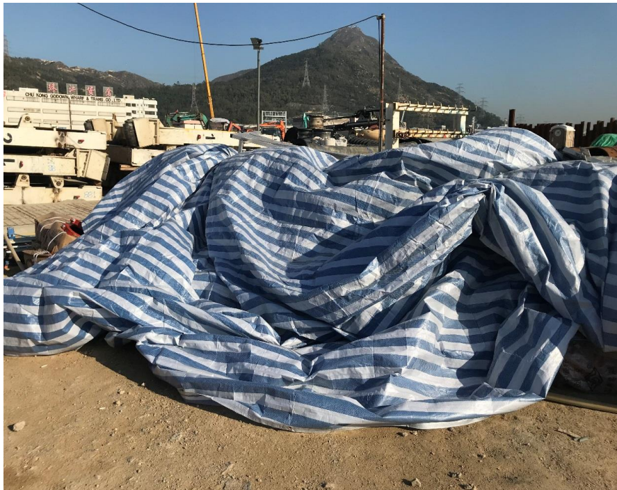
Dusty material was covered by tarpaulin sheets. (Works Area Portion N-A)
