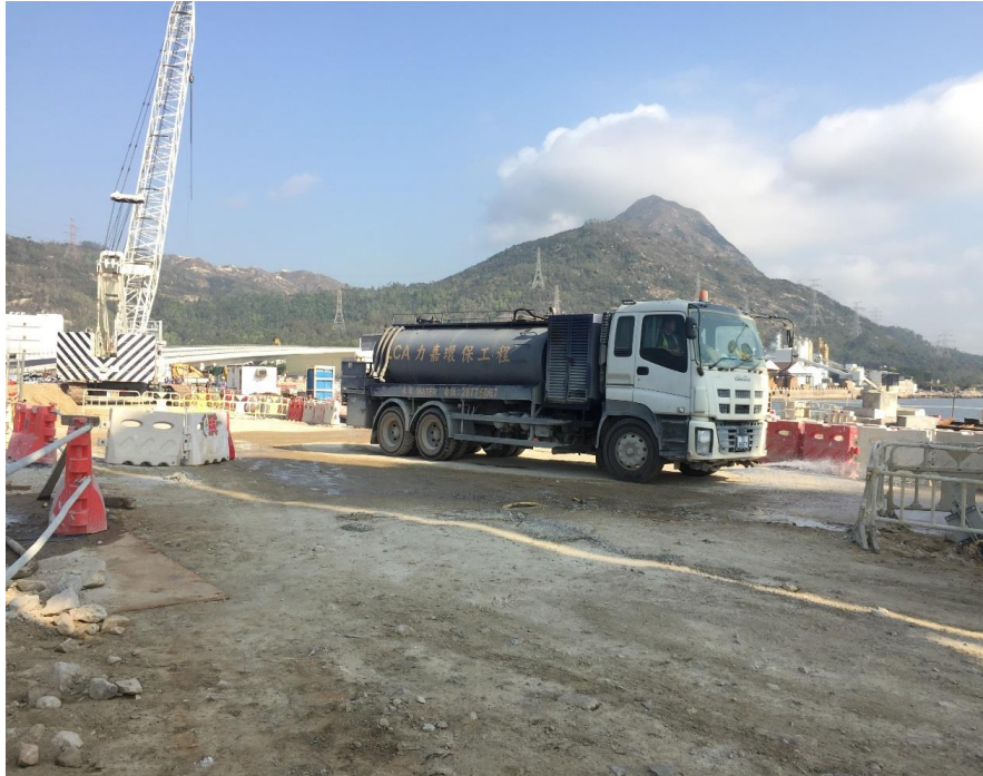
Water truck was used for water spraying to prevent dust. (Works Area Portion N-A)
