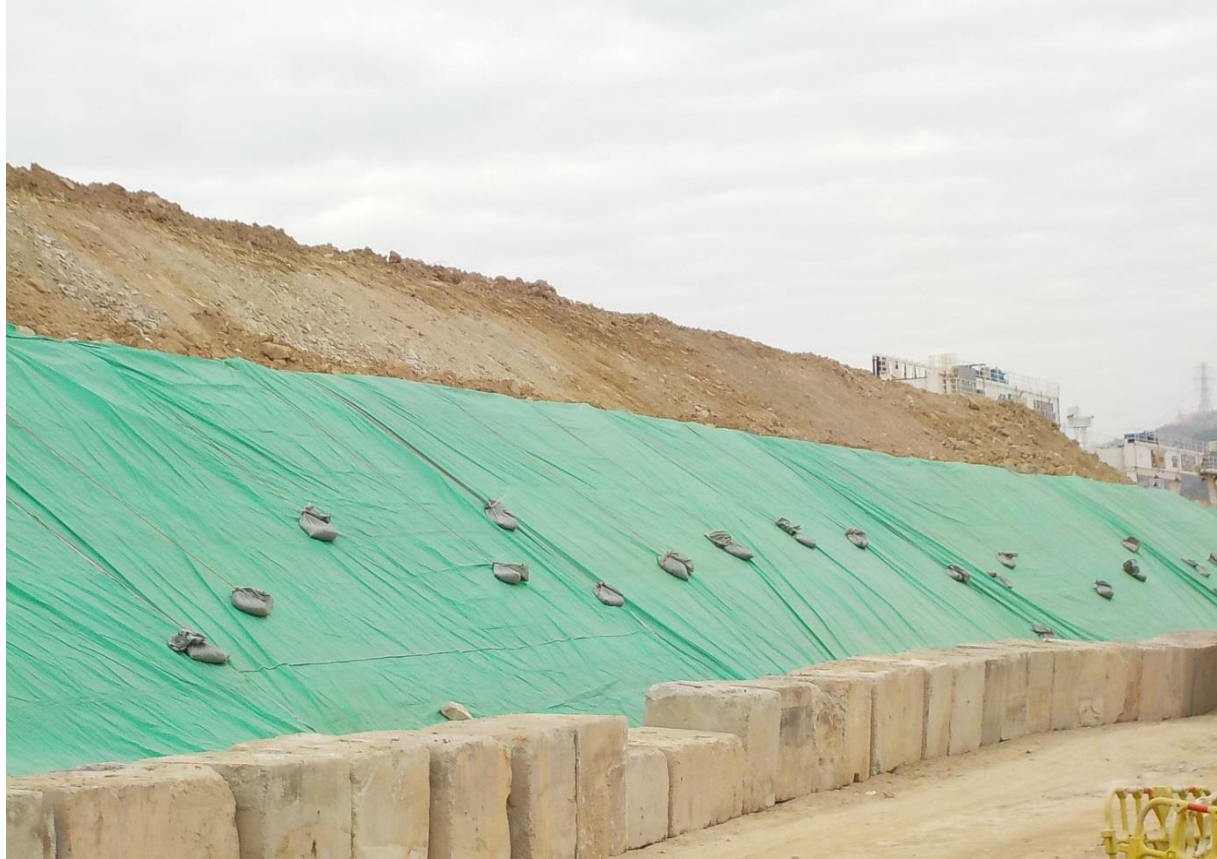
Exposed soil are covered by tarpaulin sheets to prevent dust. (Works Area Portion N-C)
