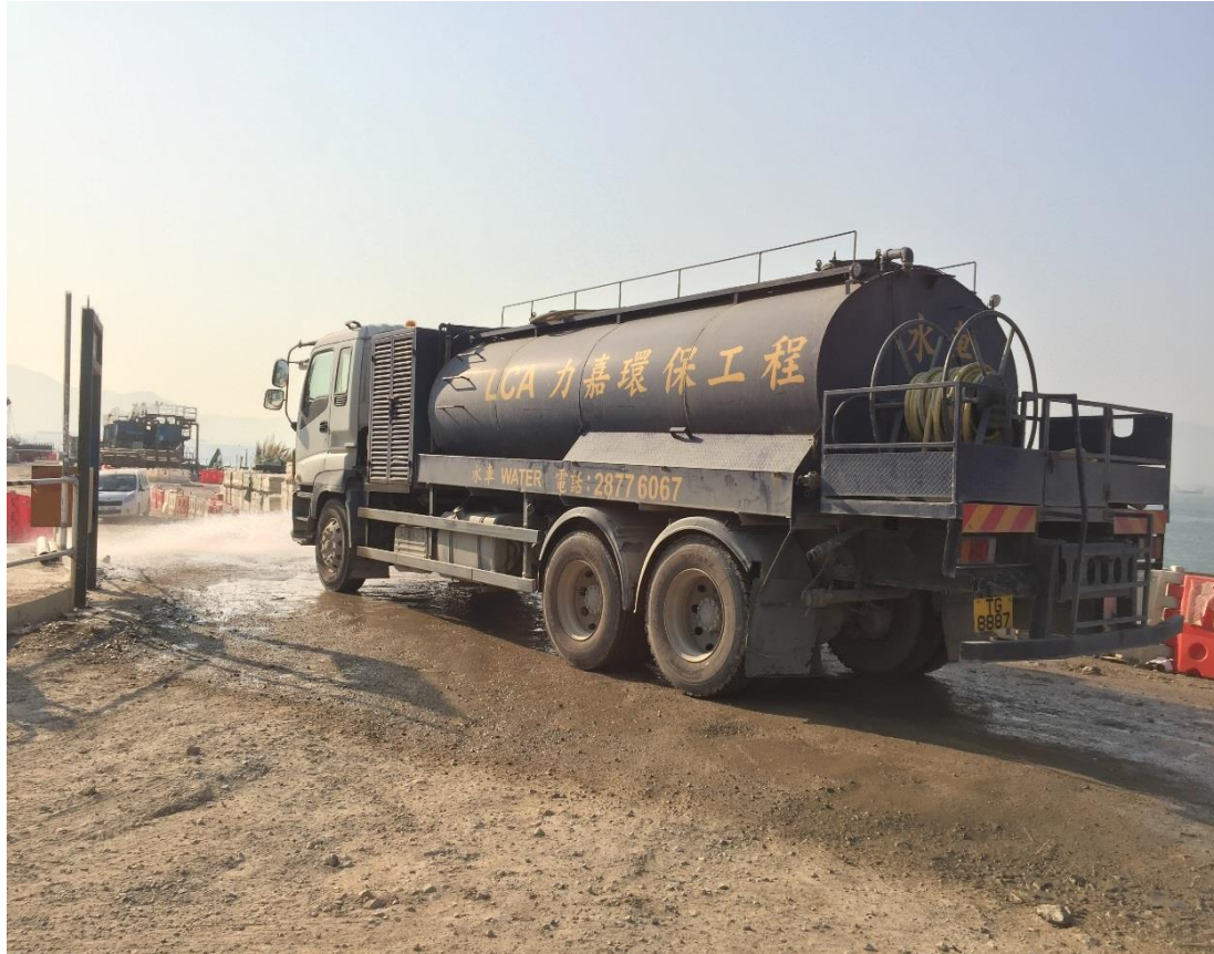
Water truck is used for water spraying at works area. (Works Area Portion N-C)
