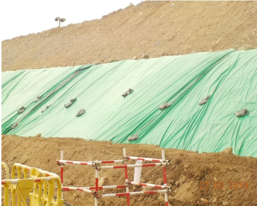
Exposed soil was covered by tarpaulin sheet to prevent dust. (Works Area Portion N-C)
