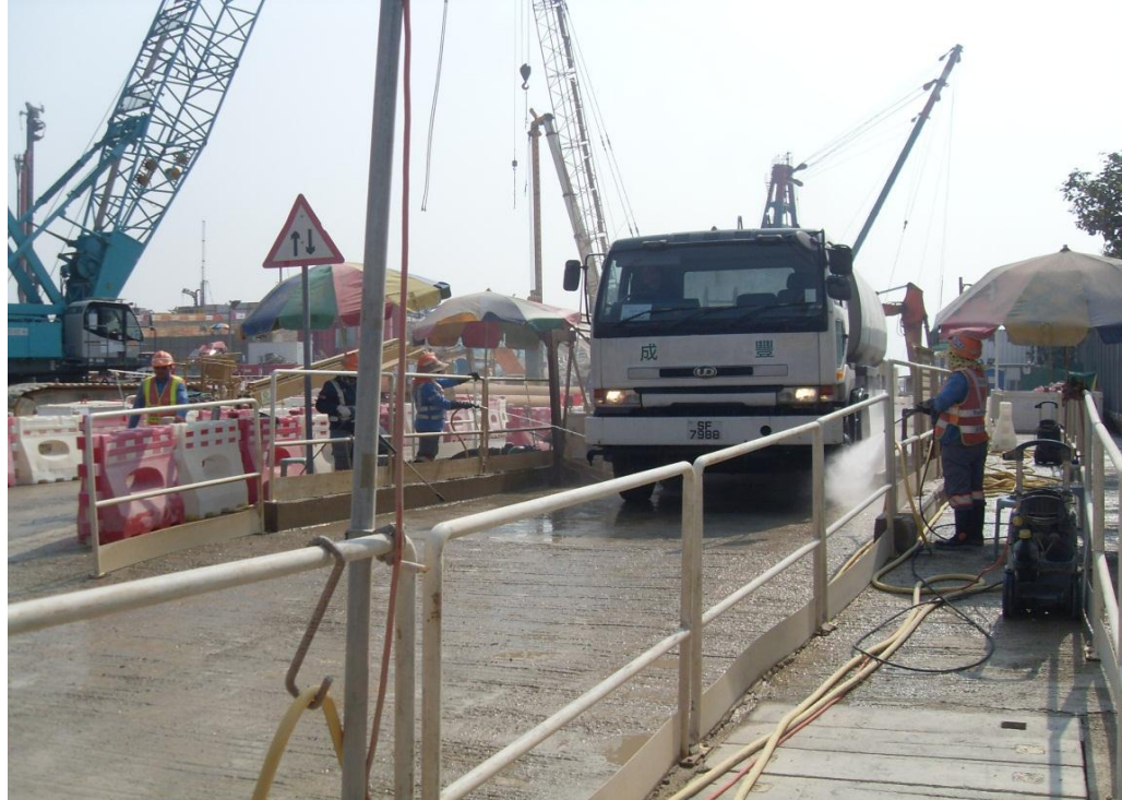
Wheel washing facilities is adequately maintained. (Site entrance at Reclamation Works Area)
