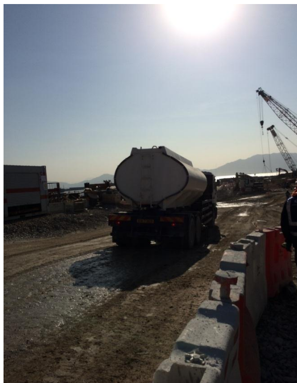
Use of water truck on exposed soil within the Project site and associated work areas. (Reclamation Works Area)
