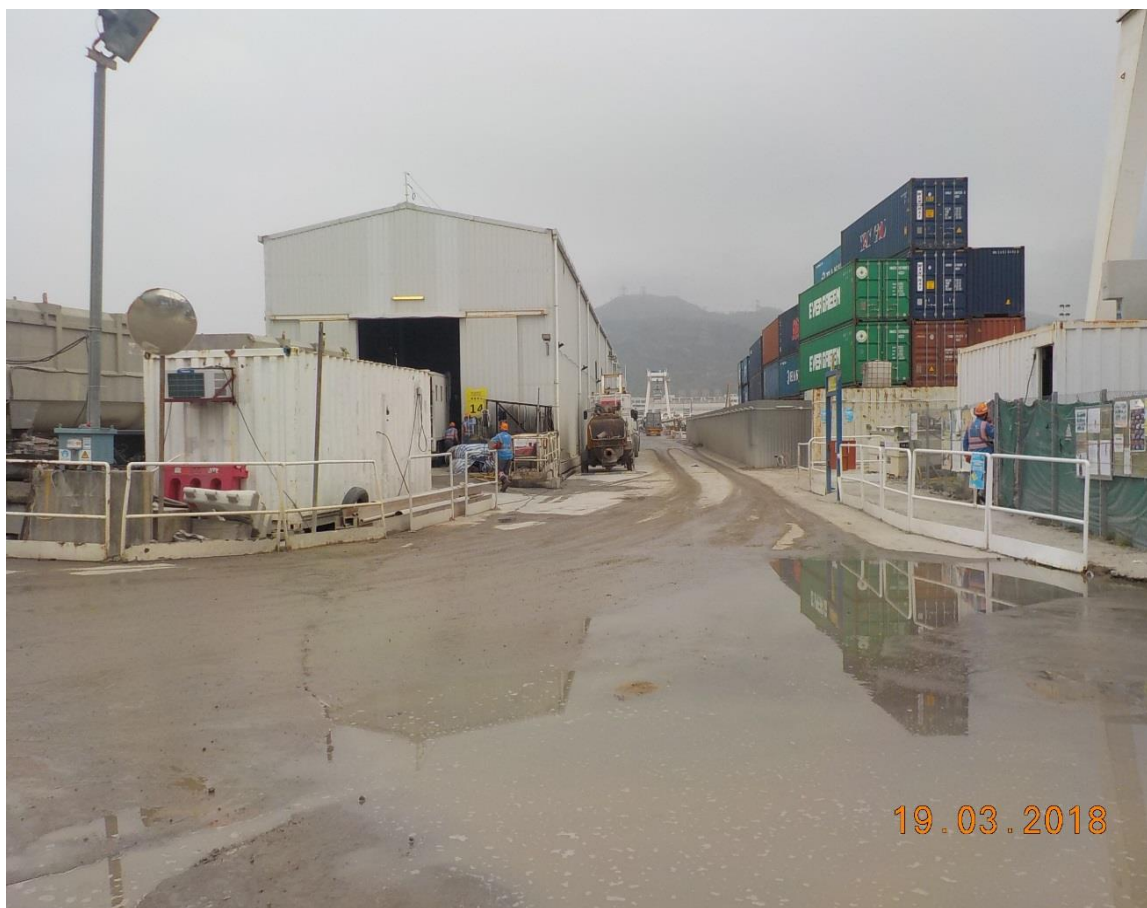
Water spraying was applied frequently on site. (Works Area Portion N-B)
