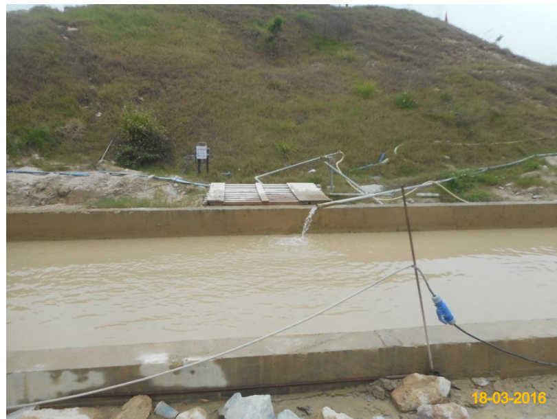
Item 4. Hydro-seeding or sheeting provided at stockpile.
