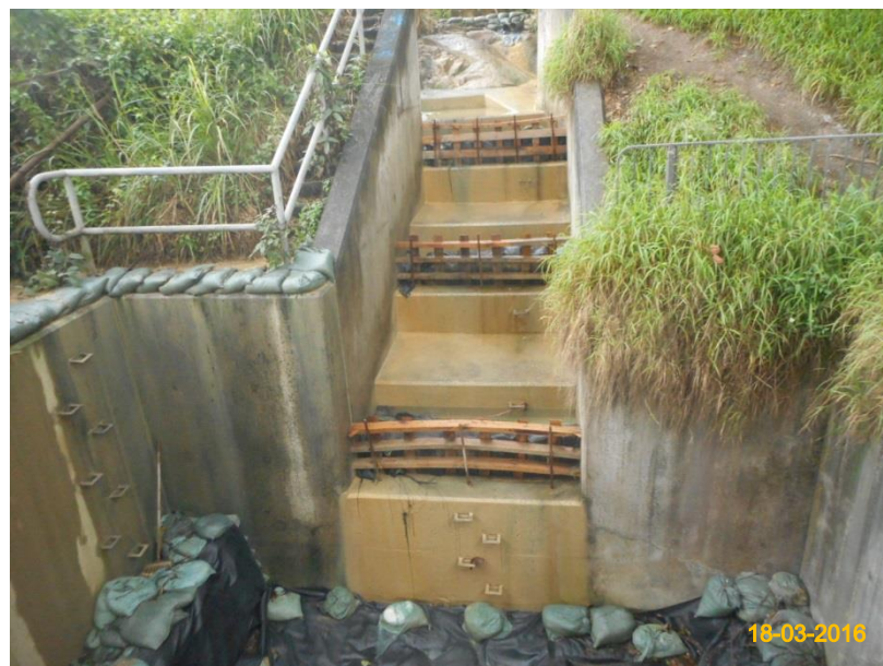
Item 7. Ensure no run-off into water body.
