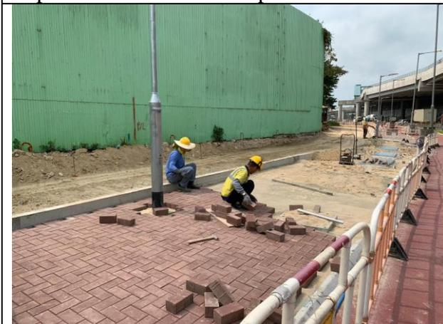
**Photo 11** Paving block works at Lung Mun Road
