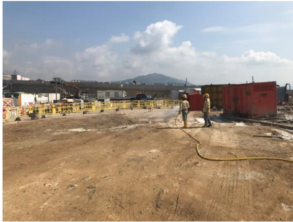
Photo 1 - Watering of unpaved roads to maintain a wet condition (31 October 2018)
