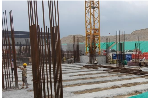
Photo 2- Building structure was conducted at works area of Customs and Excise Building (24 May 2019)
