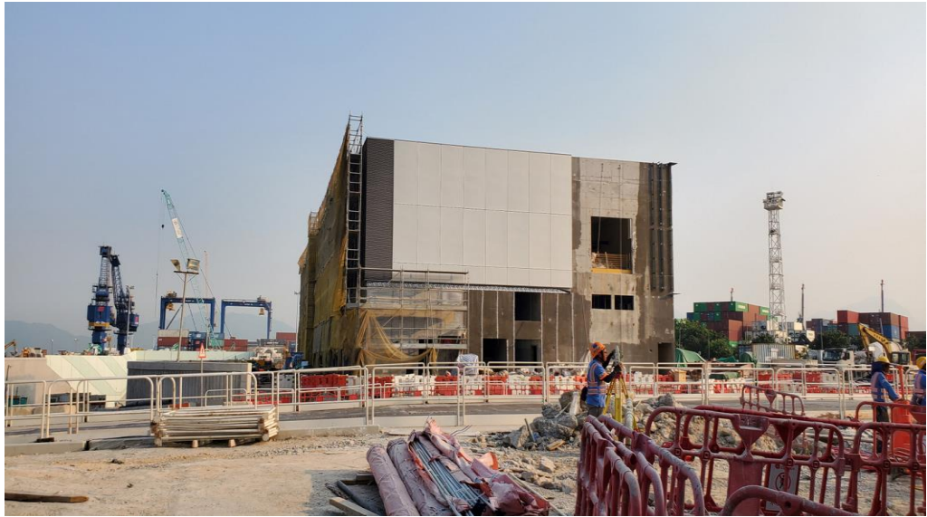
Photo 1 - Construction works at Administration Building
