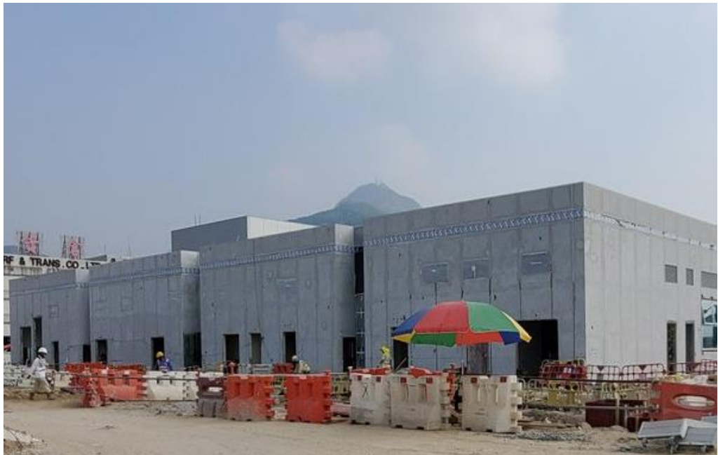
Photo 2 - Construction works at Maintenance Depot
