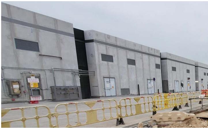
Photo 2 - Construction works at Maintenance Depot
