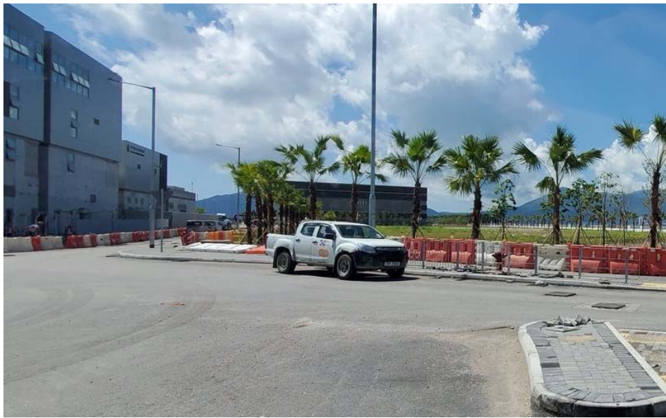
Photo 2 -North Ventilation Building
