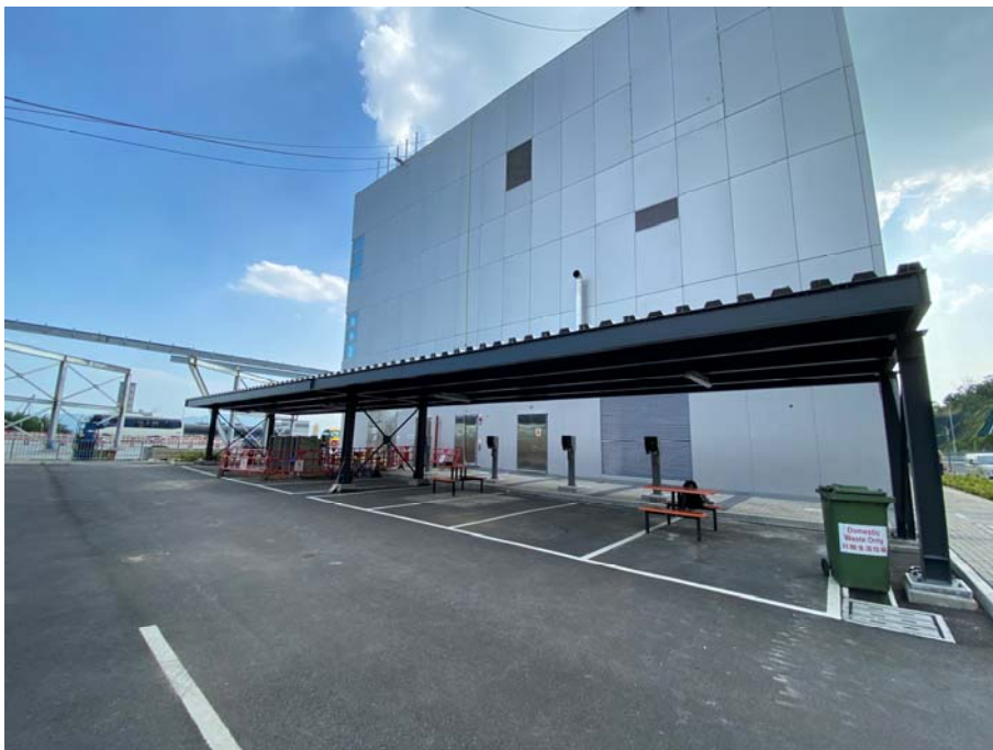
Photo 2 - Main Control Building
