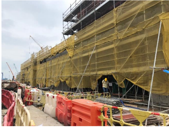
Photo 1 - Structure building at Maintenance Depot
