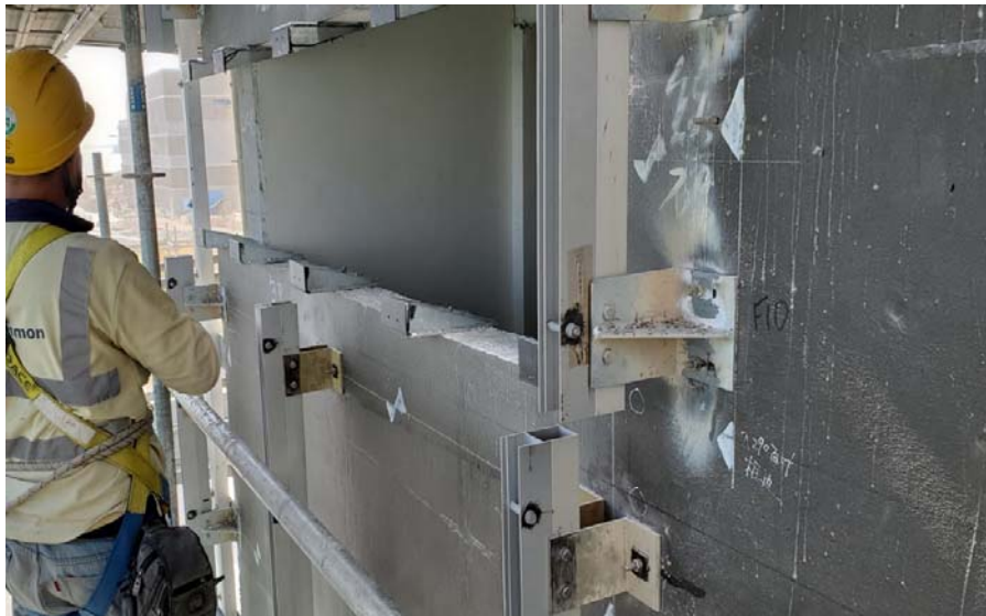
Photo 3 - Construction works at Fire Services Department Building
