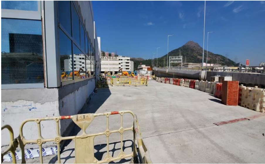
Photo 2 - Construction works at Maintenance Depot
