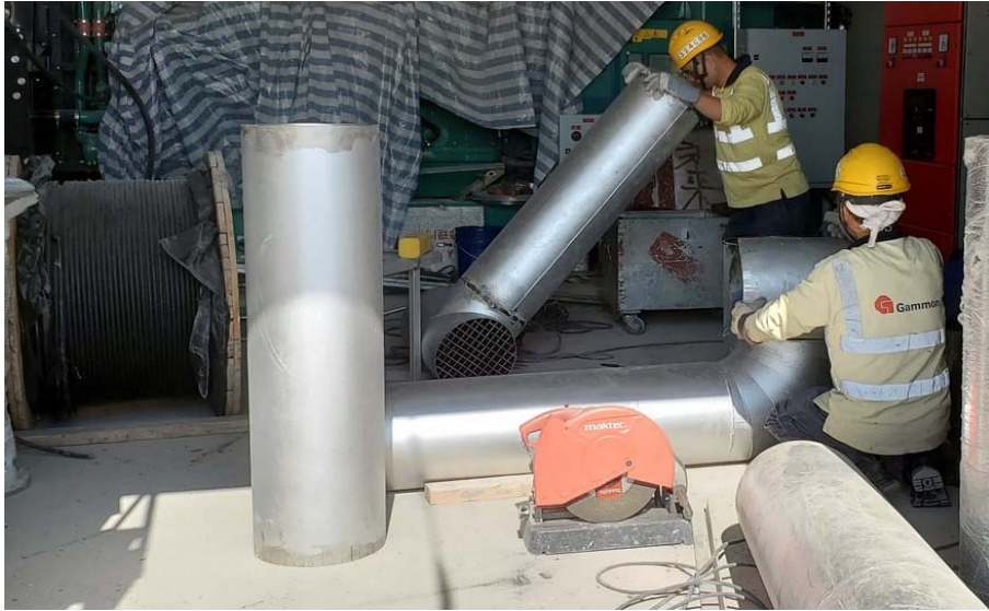
Photo 1 - Construction works at Administration Building
