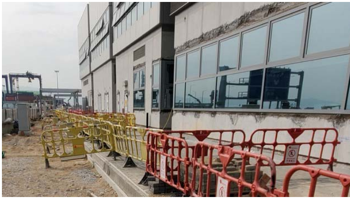
Photo 1 - Construction works at Administration Building
