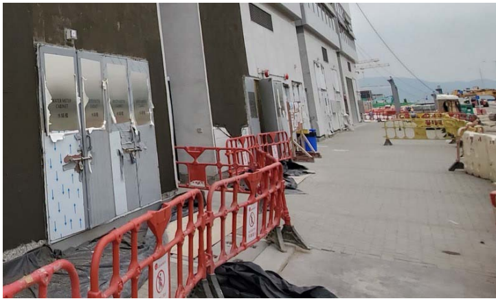
Photo 1 - Construction works at Administration Building
